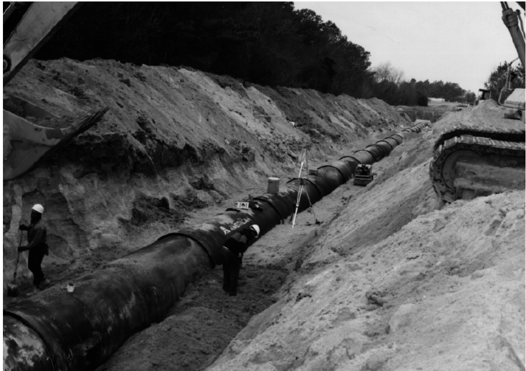
1,600mm ACIPCO Fastite Joint pipe being installed in a wastewater application.
